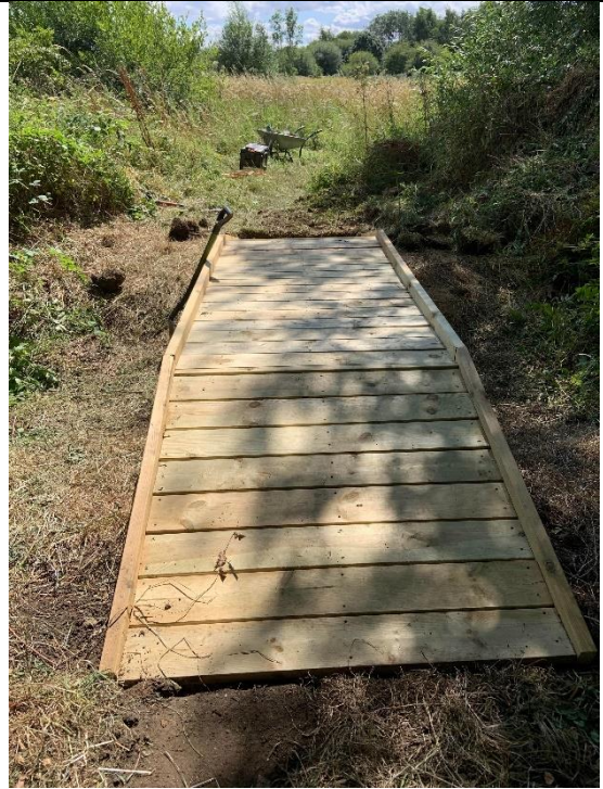
Photograph 11: Footbridge T20 in BLW T10
