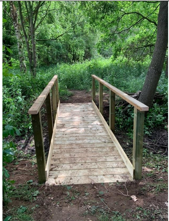
Photograph 12: Footbridge T27 over drain T6 in BLW T5
