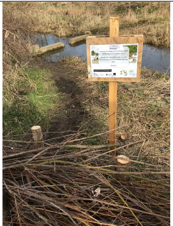
Photograph 2: New signage and brash fencing installed to deter footfall over the boundary drain T26
