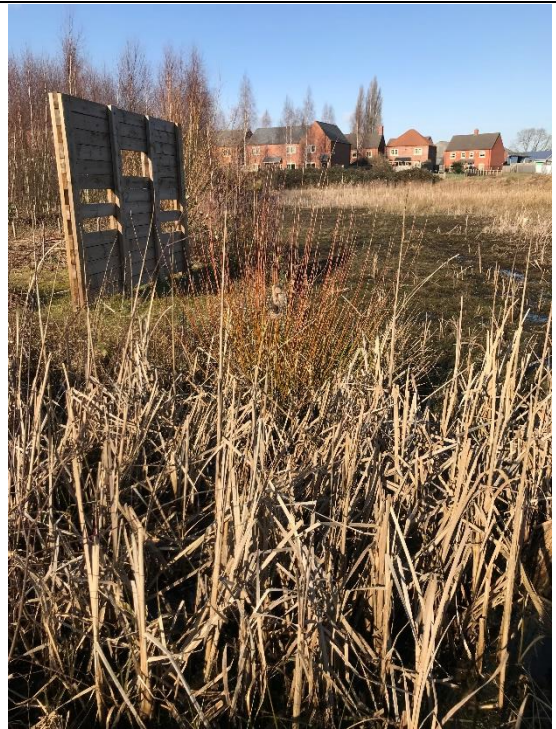
Photograph 4: View over drain T12 to bird screen and attenuation pond
