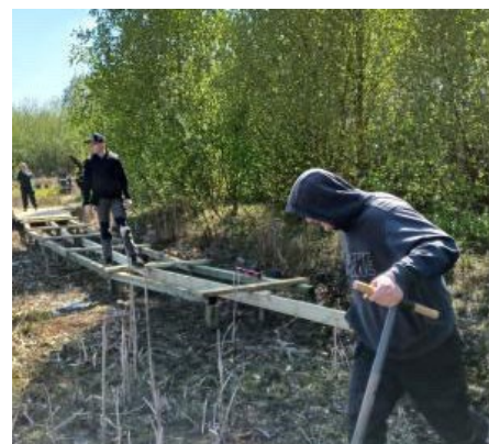
College group helping construct the boardwalk
