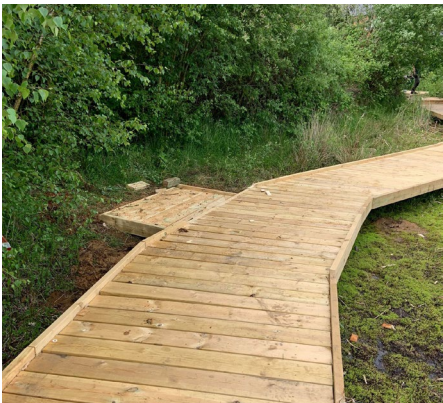
50m of boardwalk constructed
